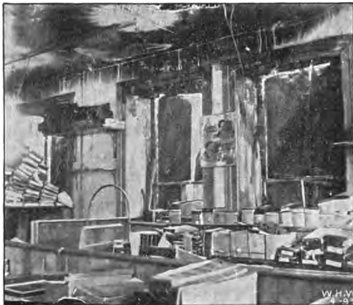
FIG. 26.—FIRE SHUTTERS DESTROYED—FIRE HELD IN CHECK BY AUTOMATIC SPRINKLER.
