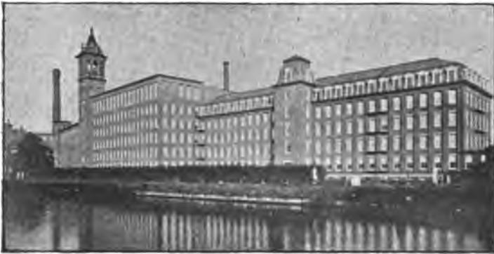
FIG. 11.—MILL WITH SLOPING MANSARD ROOF. (Atlantic Mills, Lawrence.)
