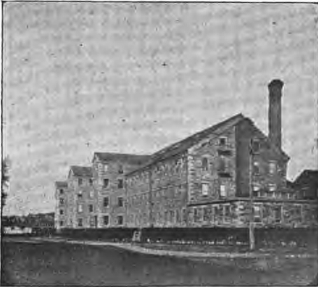
FIG. 8.—FACTORY WITH "BARN ROOF," (Erected 46 Years Ago.) (Everett Mills, Lawrence, Mass.)
