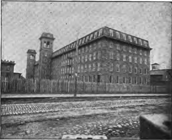
FIG. 12.—MILL WITH FLAT MANSARD ROOF. (Merchants' Mfg. Co., Fall River.)
