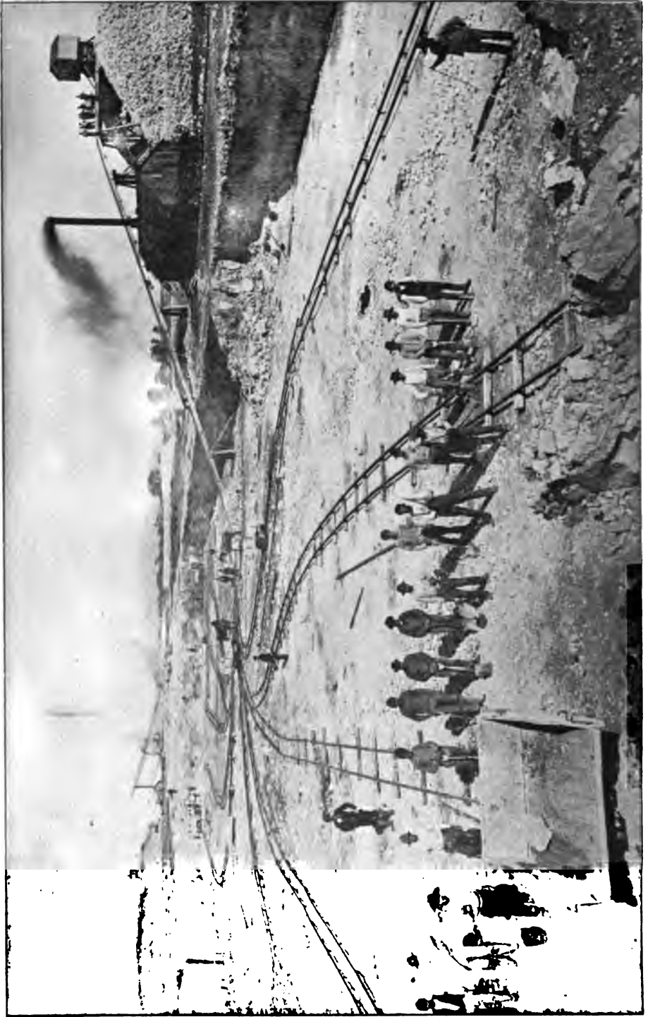
PLATE IX.—DRAINAGE CANAL AND WATERWAY IN ROCK. FULL WIDTH AND ONE THIRD REQUIRED DEPTH.
