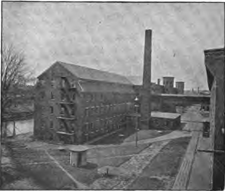
FIG. 5.—A NEW HAMPSHIRE MILL WITH FACTORY ROOF, ERECTED SIXTY YEARS AGO. (Indian Head Mill, Nashua.)
